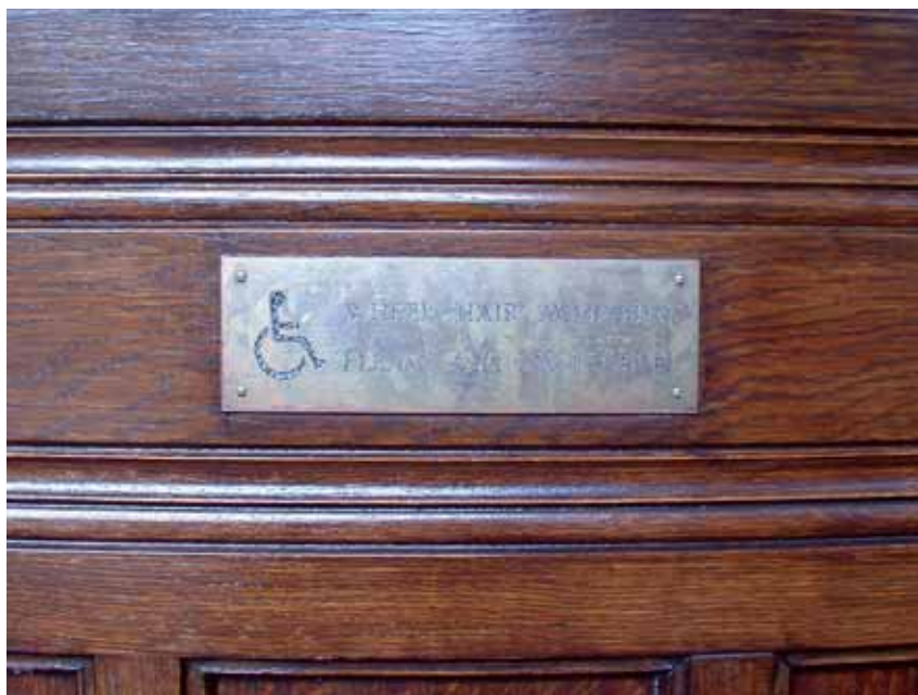
Signs must be maintained in order to remain accessible. This sign telling wheelchair users that they can ring for assistance is virtually unreadable through lack of maintenance.
